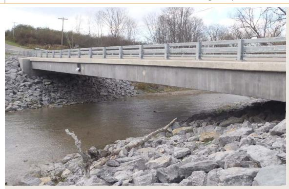
DiDonato provided comprehensive engineering services for the replacement of the Ashford Bridge No. 24 on Thomas Corners Road over Buttermilk Creek. This project involved the removal of the existing structure and realignment and replacement with a new, longer structure and improvements to the creek to provide enhanced hydraulic characteristics through the new structure.
